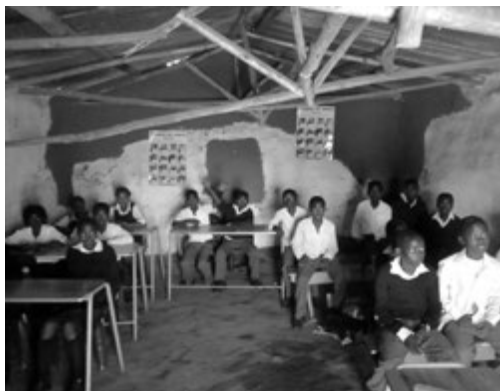
Photo A (taken 25 February 2013) – the inside of the mud structure church which functions as a grade 6 classroom at Samson SPS. The trusses are collapsing and the roof leaks badly.
